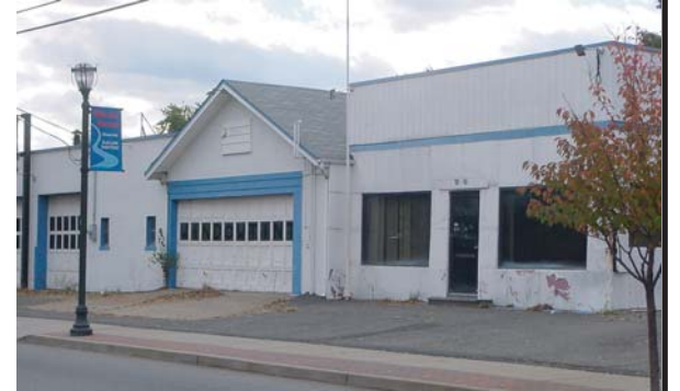
Interstate Glass, 10-16 River Road, is under development
