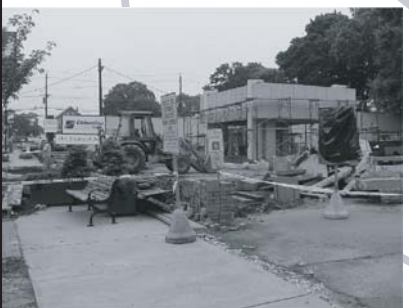
Columbia Bank is currently constructing three drive-thru lanes and an ATM.
